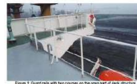
Figure 1. Guard rails with two courses on the open part of deck structure Source: IMO SDC 10/11
