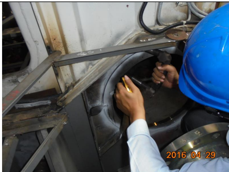
磁粉檢驗法 (Magnetic Particle Inspection)
